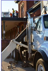
Canopy roofing work underway on Aug 24, 2013, at Jackson depot.
