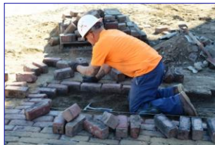
Tim Gaddis of Drew Mechanical of Waterford, installs a flush-mounted storm drain in the parking lot in front of the depot.
