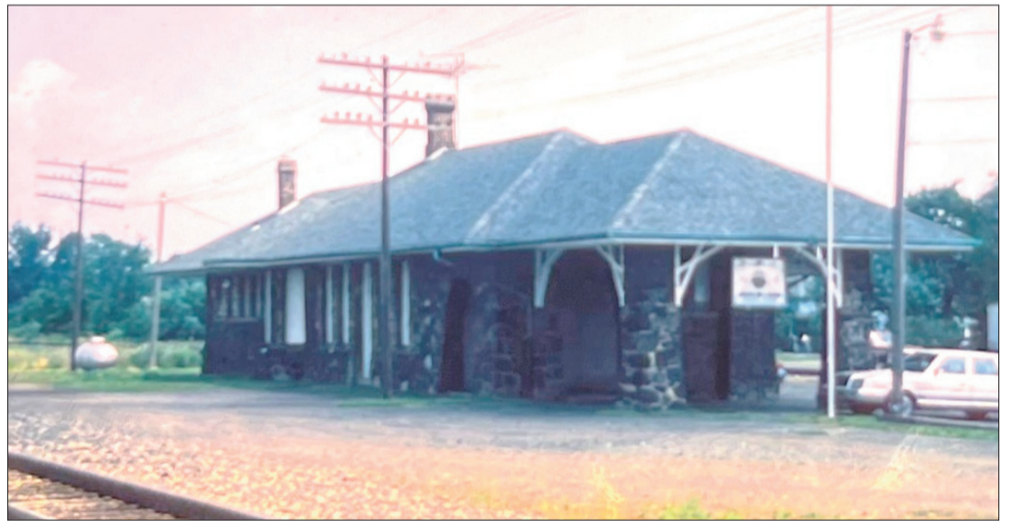
Former Michigan Central Station in Wyandotte on Oak Street. This station is located between the north and south bound Conrail tracks, which are about 125 feet apart at this location. Both tracks could be served by this station.
