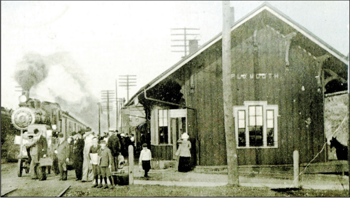
Photo from circa 1910 of the Pere Marquette station building in Plymouth on Starkweather Street. The building remains in place as an ice cream shop.
